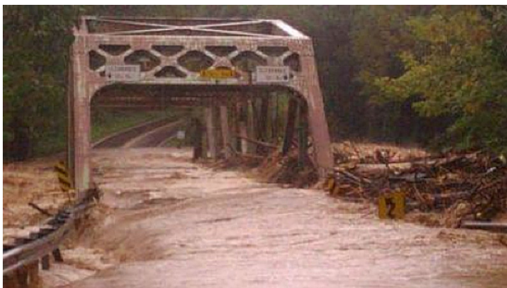
Bridge in Mehoopany, PA (Wyoming County) taken out by Hurricane Irene.
